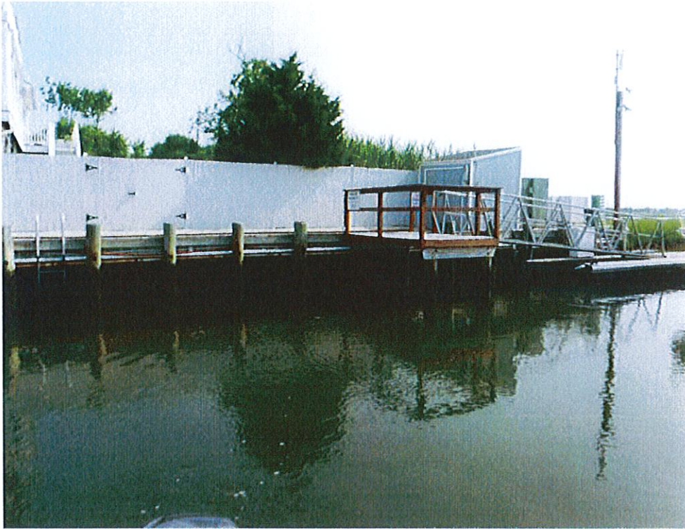
Photo 9: View of bulkhead east of C Dock
