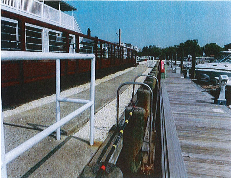
Photo 26: Looking south along the bulkhead and club house deck
