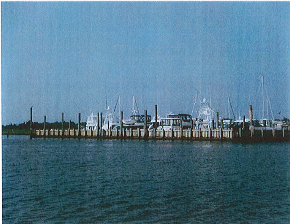
Photo 2: Overall view of northern section of new wave screen
