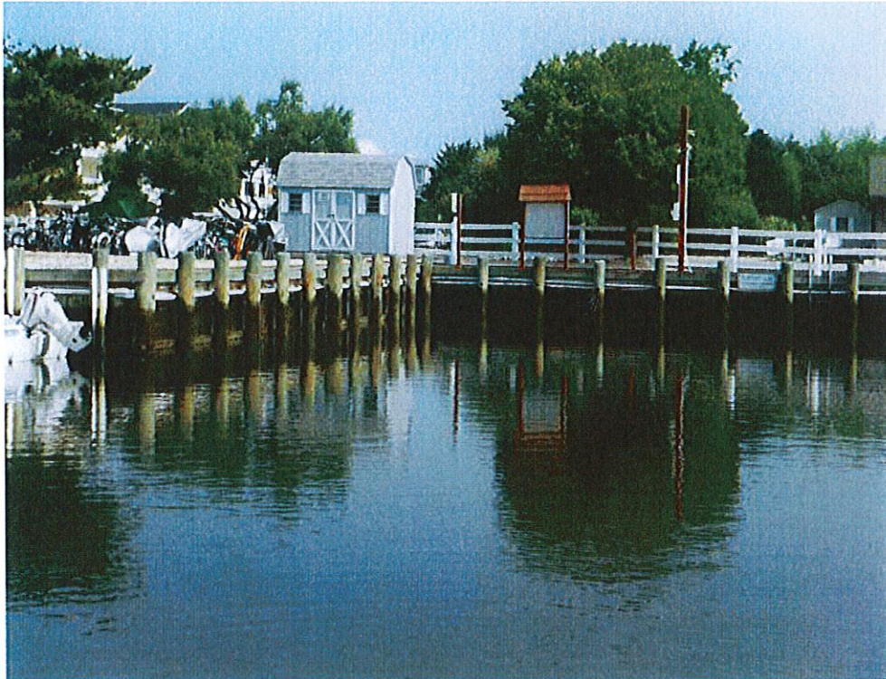
Photo 15: View of the northwest corner of the bulkhead
